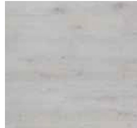
BATH 3 FLOOR MANNINGTON NEXCORE (HOUSTON CONCRETE)
